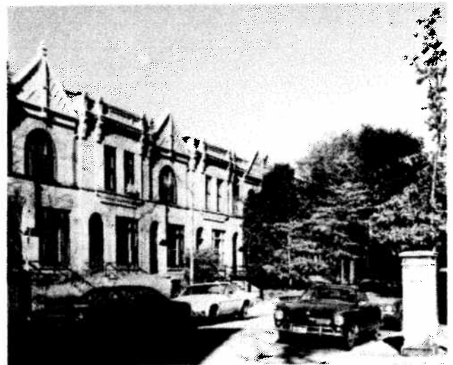
A view of the west side of Crilly Court. These simplified Queen Anne style row houses were constructed in 1885 as part of Daniel Crilly's project to develop the entire 1600 block between North Park Avenue and Wells Street. The unique character of the block has been retained and today the Crilly buildings are a particularly popular place to live. (Barbara Crane, photographer)
